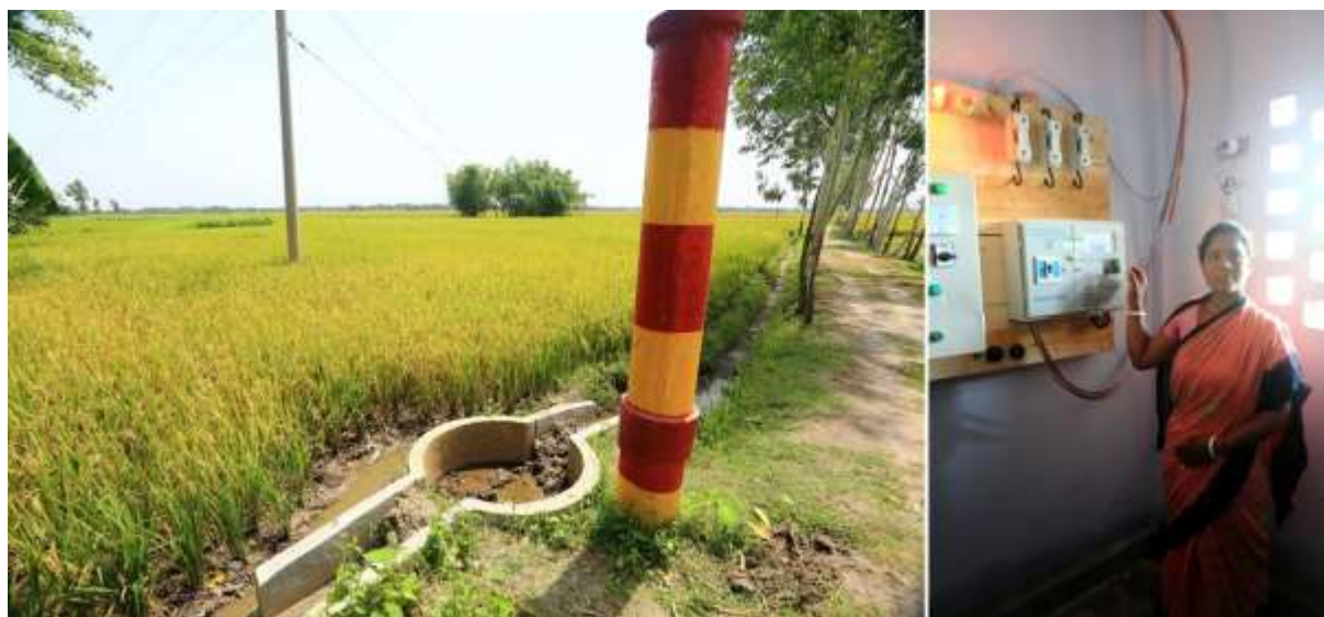
Figure 20. A distribution gully to which water is pumped from the DTW (left), and a women operating the electric card system (right).
