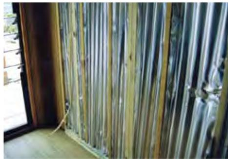
Two forms of insulation are used – radiant (aluminium foil backed felt) and bulk insulation to address extreme solar conditions of the site.
