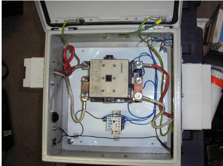
**Figure 5.3:** Photo of Contactor Box
