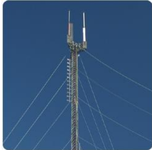
Figure 5-2 Image Showing Guy Wire Placement on Radio Tower (Zhejiang Guanming Power Transmission Material Corp. 2016)
