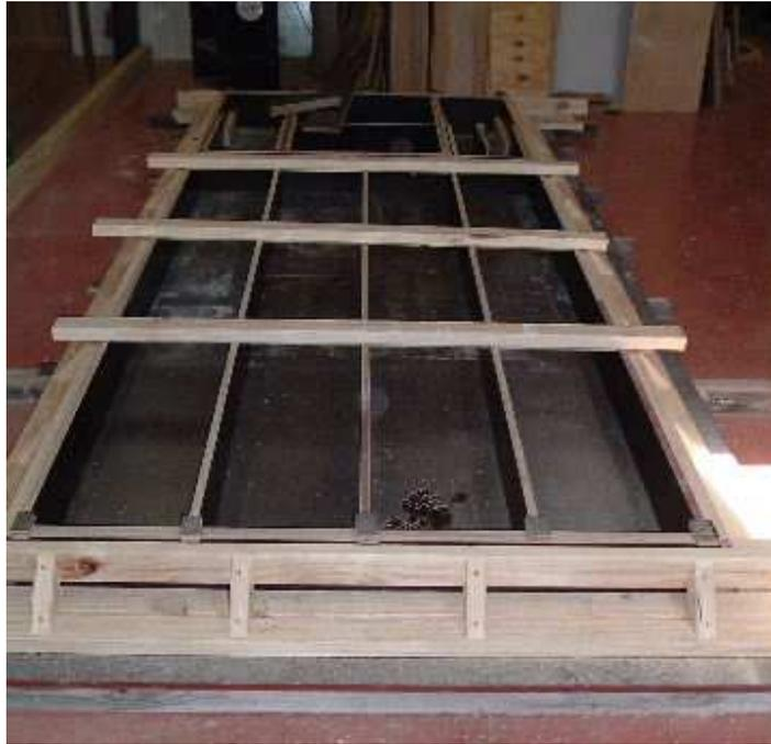
**Figure 4.1:** Formwork to Cast Beams
