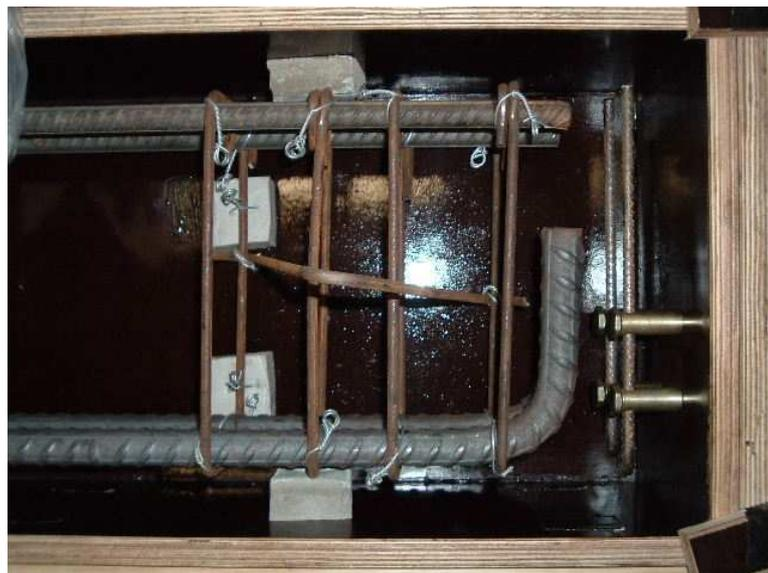
**Figure 4.3:** Positioning of Reinforcement Cages
