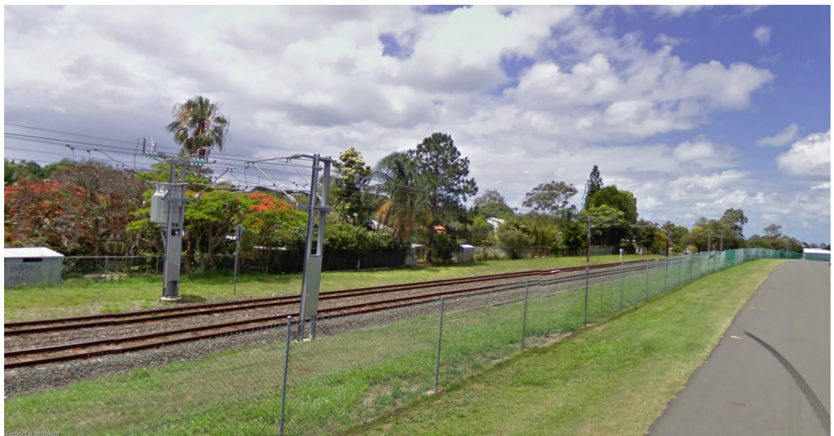
Figure 31: Existing Cleveland Rail Line Elevation Looking East (Google Maps)
