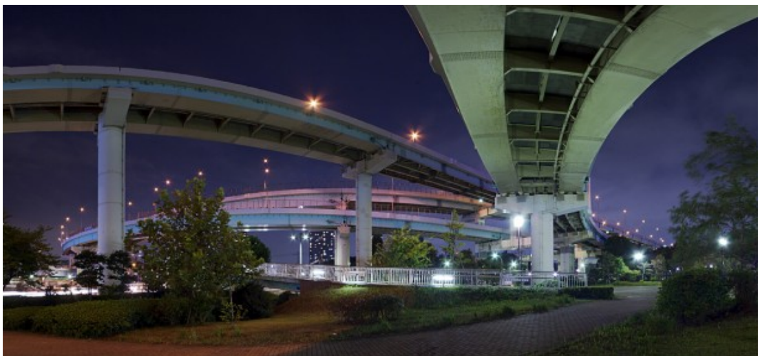
Figure 6: Looking from the Side, Elevated Highways in Bangalore, India ( www.aldafla.com )
