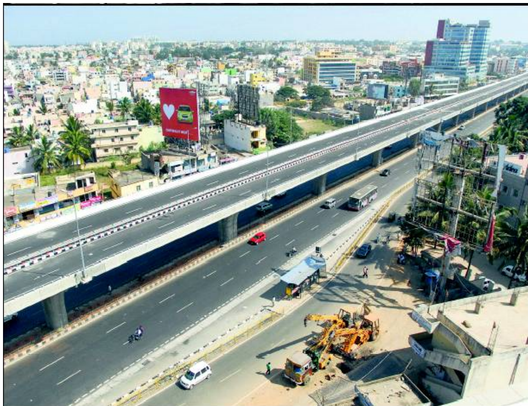
Figure 10: Top View, Elevated Highways in Bangalore, India
