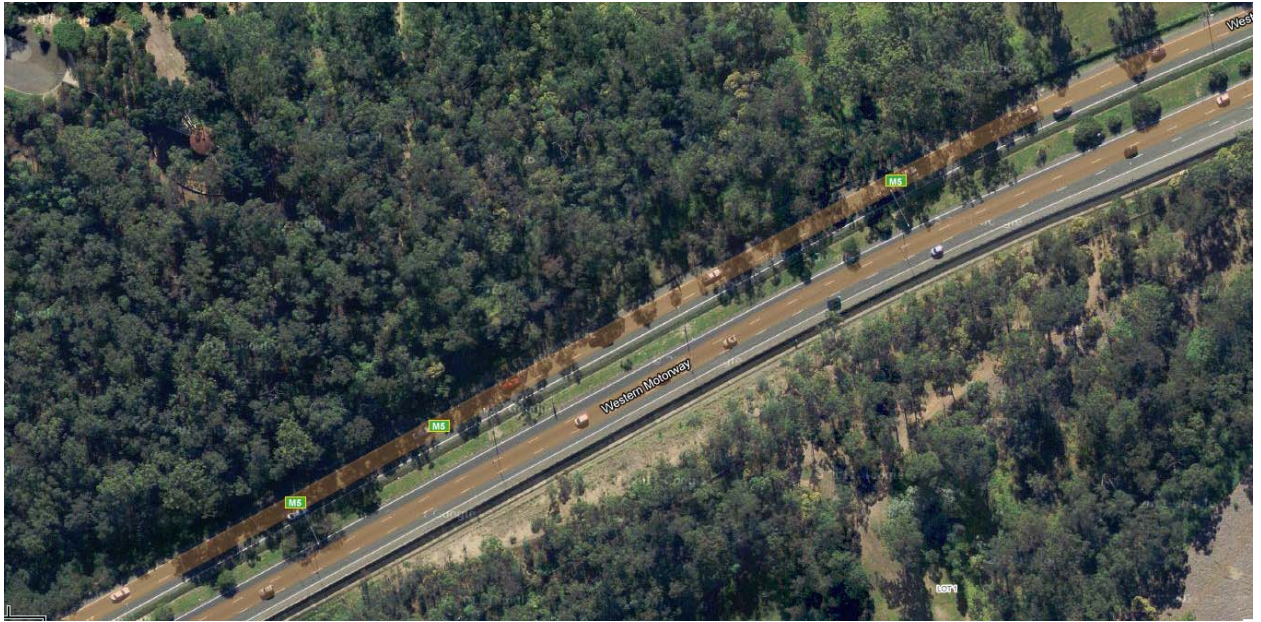
Figure 53: A Portion of the Existing Western Freeway Plan View (Google Maps)
