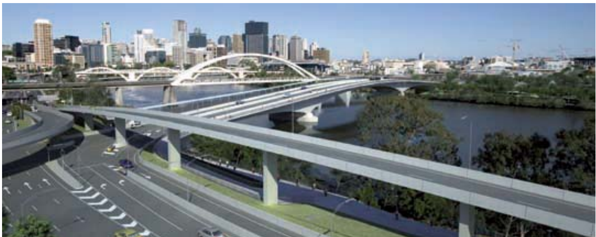
Figure 16: Newly-Constructed Go-Between Bridge and Coronation Drive Flyover - Milton, Brisbane QLD (*7.BCCTP)
