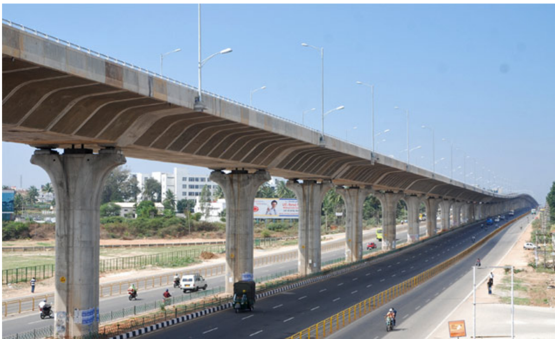
Figure 8: Elevation View, Elevated Highways in Bangalore, India ( www.aldafla.com )
