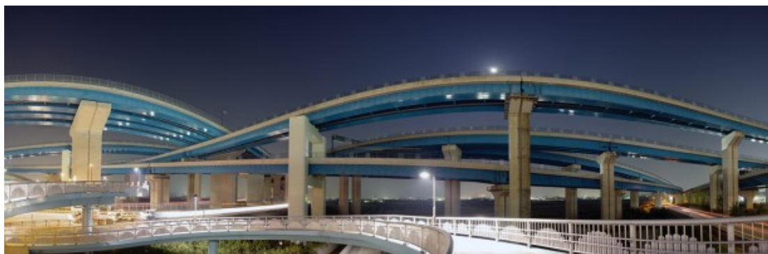
Figure 4: Overall View, Elevated Highways in Japan ( www.aldafla.com )
