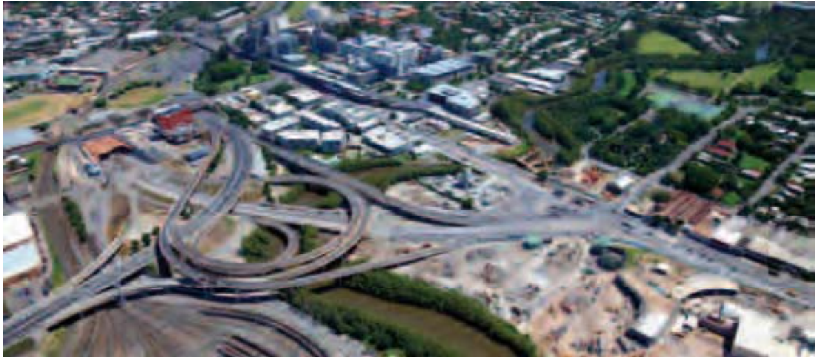
Figure 15: Construction of Clem7, Airport Link and Inner City Bypass - Brisbane, Australia (*8.SEQIPP)
