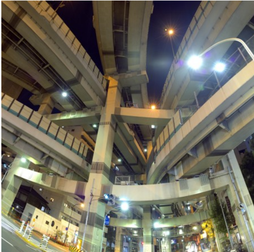
Figure 5: Looking to the Top, Elevated Highways in Japan ( www.aldafla.com )
