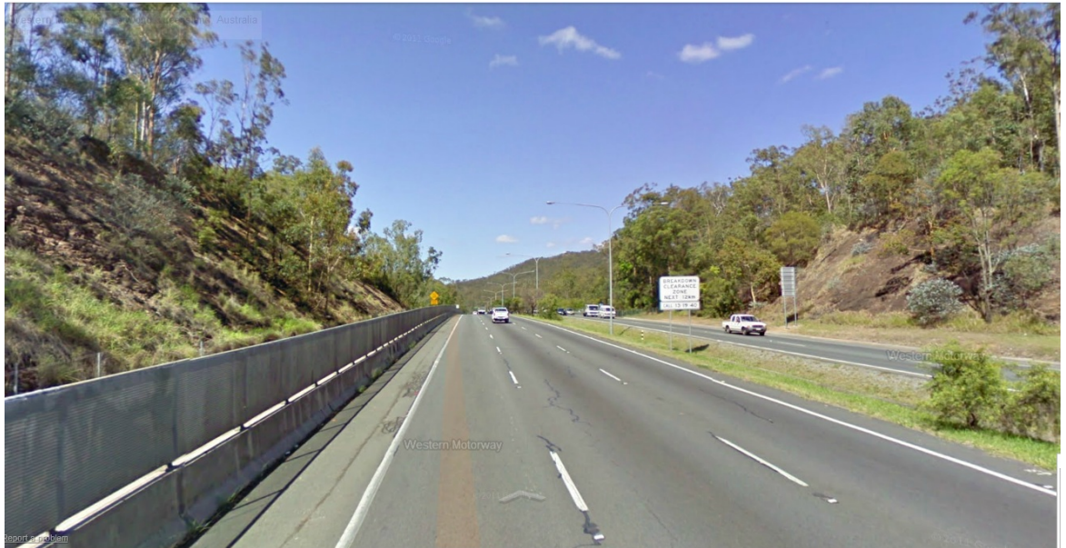
Figure 54: Existing Elevation View of the Western Freeway
