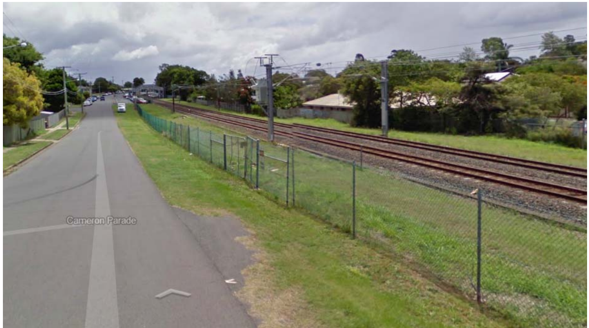
Figure 30: Existing Cleveland Rail Line Elevation Looking West
