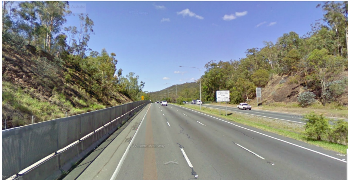
Figure22: Existing Western Freeway Elevation View Looking South (Google Maps)
