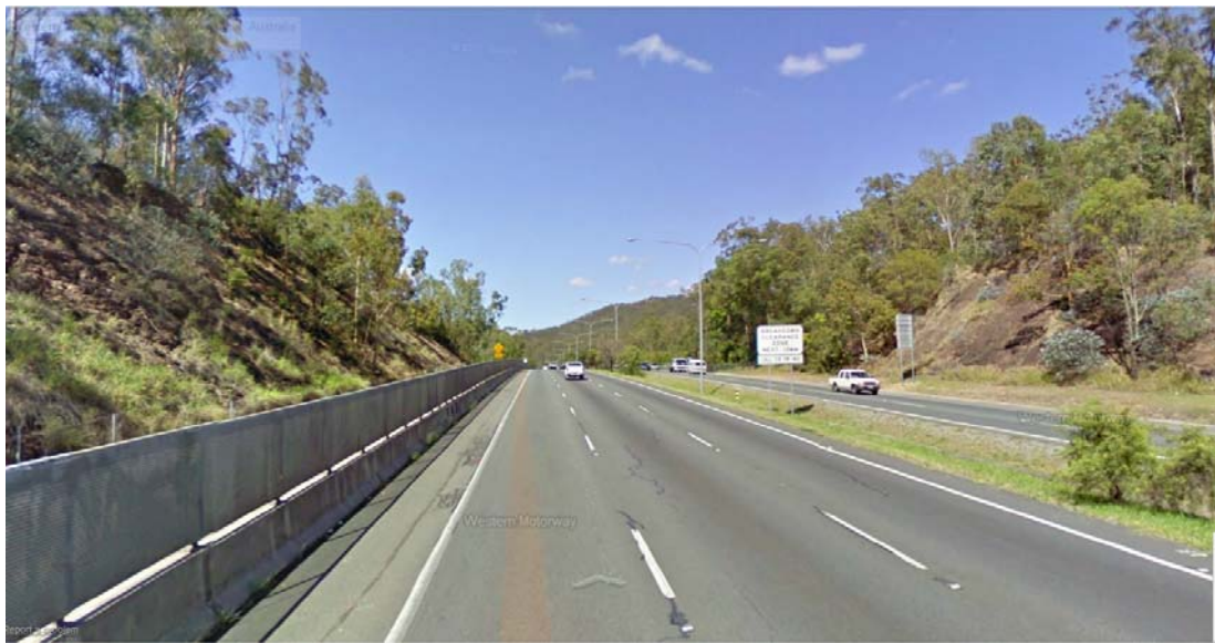
Figure 1: Existing Western Freeway Elevation, View Looking South (Google Maps)
