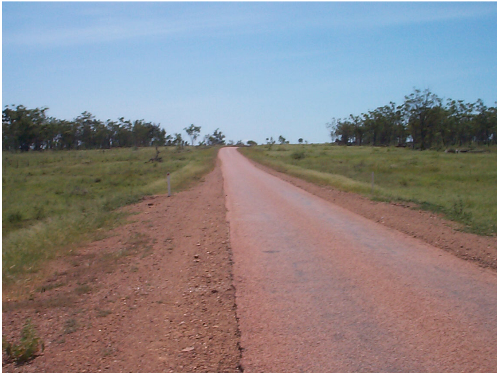
Figure 2.1 Narrow pavement width on the GDR
