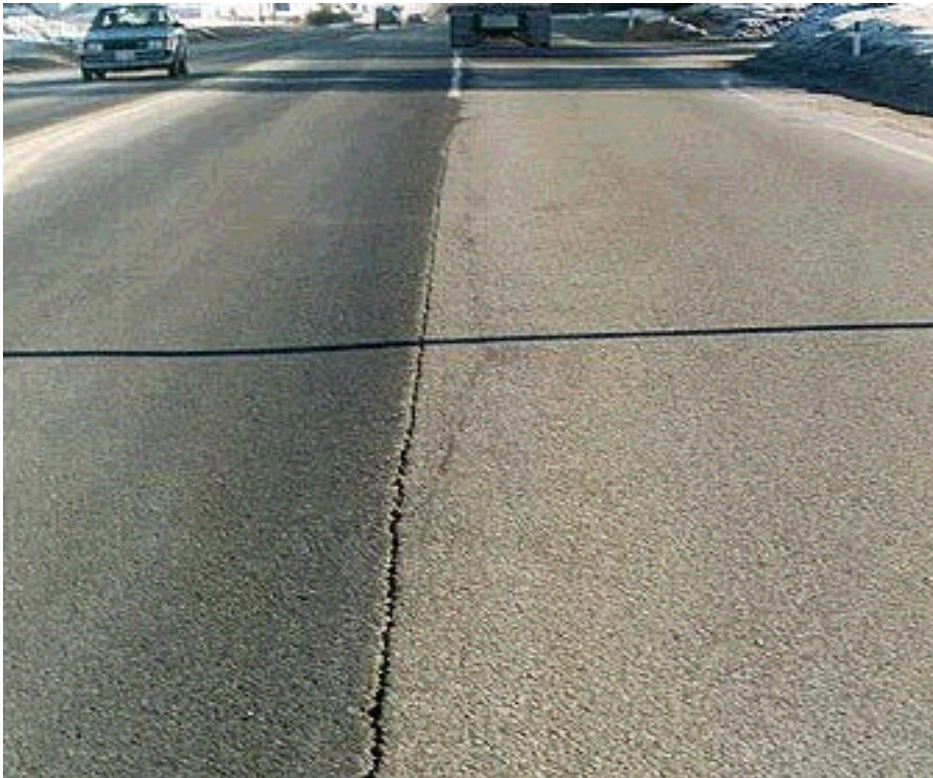
Figure 2.11 – Joint cracking due to poor joint location and construction practices
