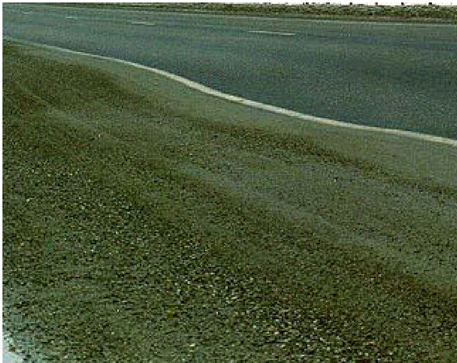
Figure 2.14 – A depression in the shoulder of a road, probably due to local moisture entry resulting in weakness of the pavement and subgrade
