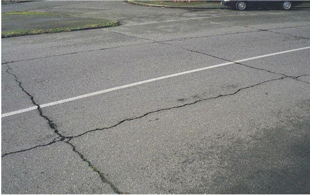
Figure 2.7 – Joint reflection cracking on an arterial road
