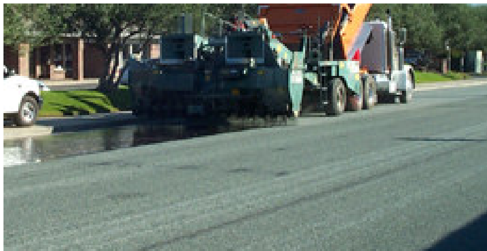
Figure 3.27 – Aggregate being placed onto top of freshly sprayed bitumen during a reseal
