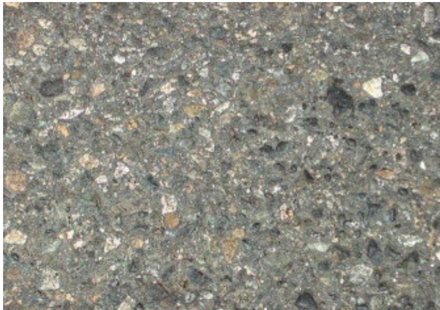
Figure 2.16 – Polishing of a surfacing. There seems to be a lack of surface texture, but no excess binder.
