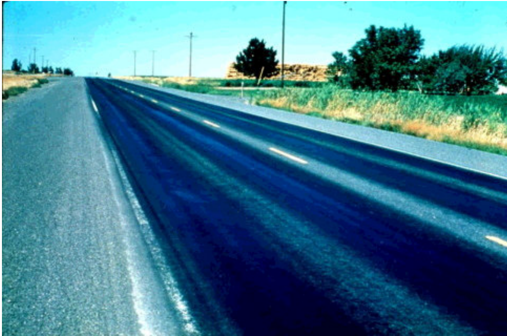
Figure 2.4 – Heavy bleeding in a spray seal
