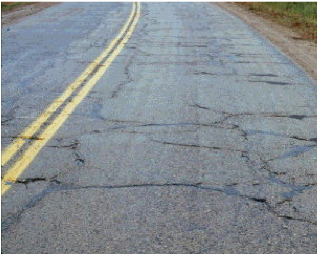
Figure 2.6 – Block cracking:
