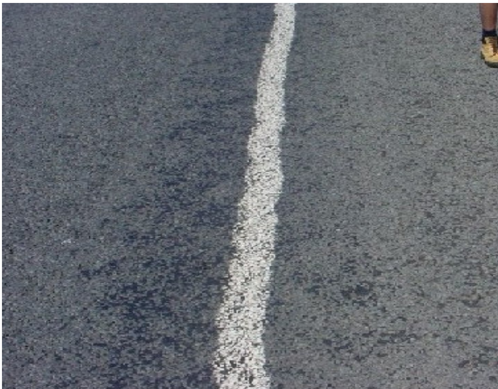
Figure 4.3 – Wavy edgeline: a) A view along the length of the job b) A closer view
