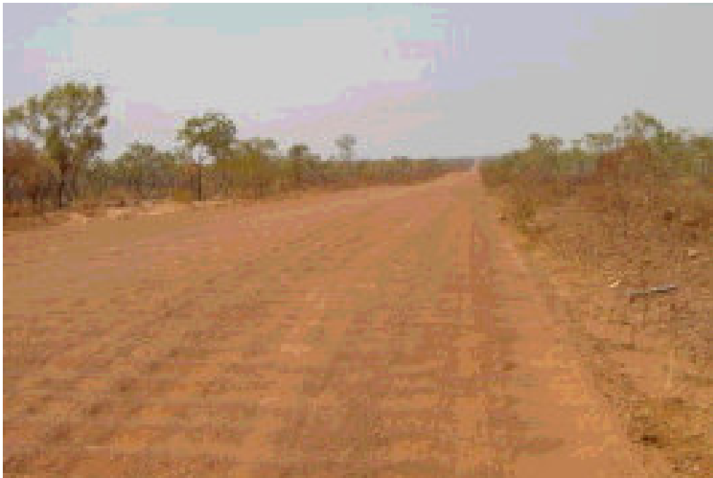
Figure 2.5 – Corrugations on a low volume road in Outback Australia
