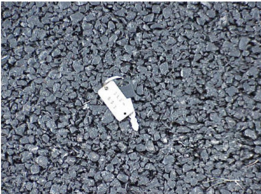
Figure 3.37 – A view of a Stone Mastic Asphalt surfacing, illustrating the high proportion of large particles present in the structure
