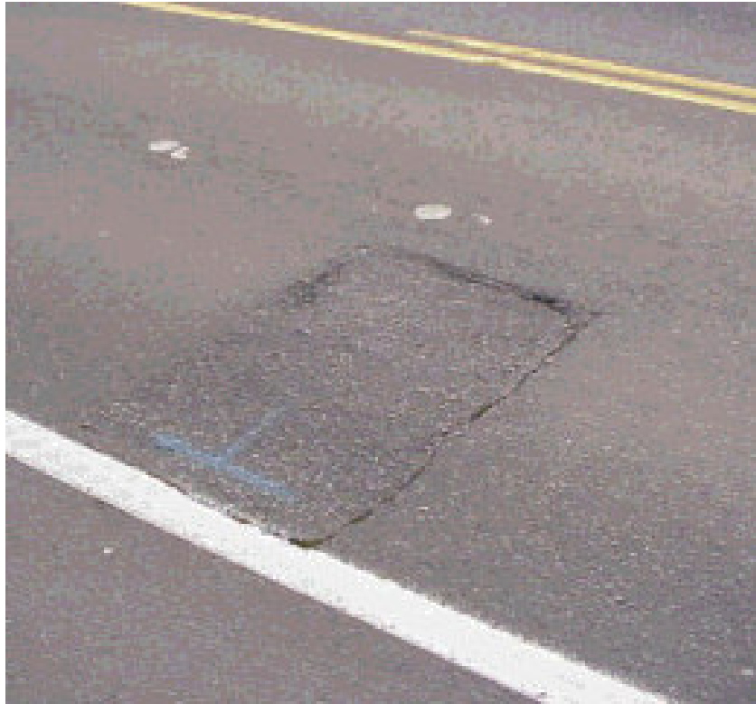
Figure 2.15 – A patch placed over an area of localised pavement distress
