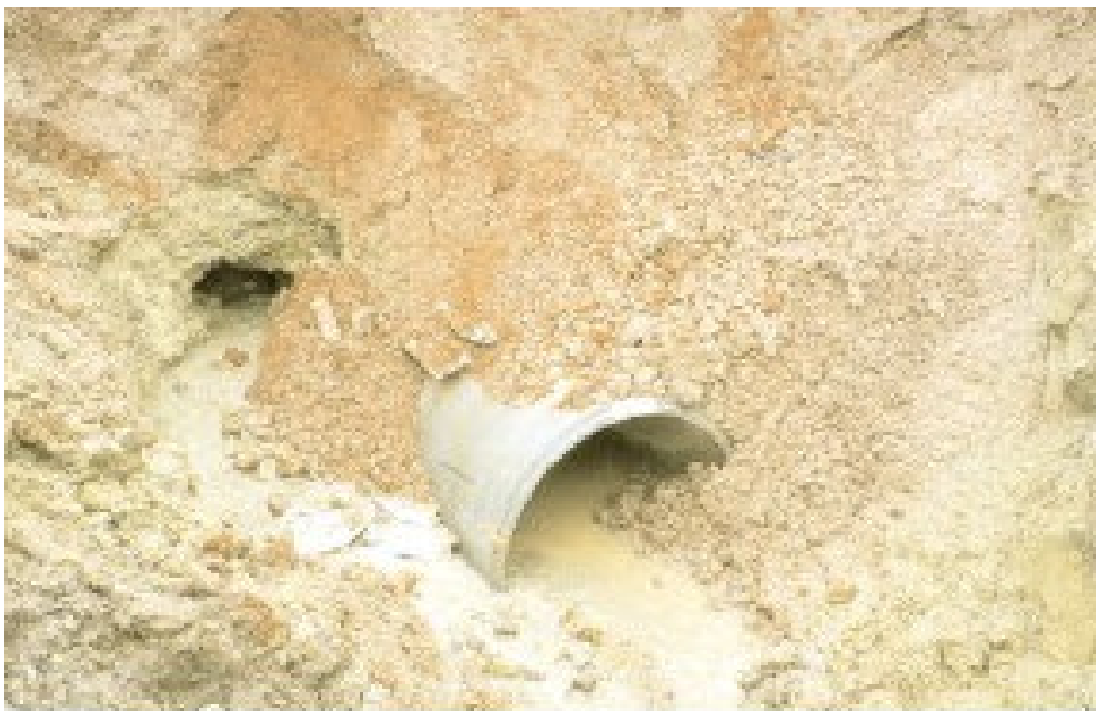
Figure 3.2 – Problems with the drainage system: a) A culvert blocked by vegetation b) A culvert that no longer functions effectively
