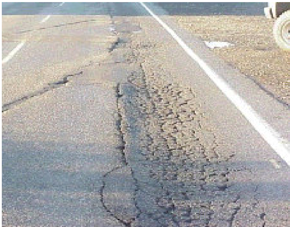
Figure 2.9 – Fatigue/structural cracking:
