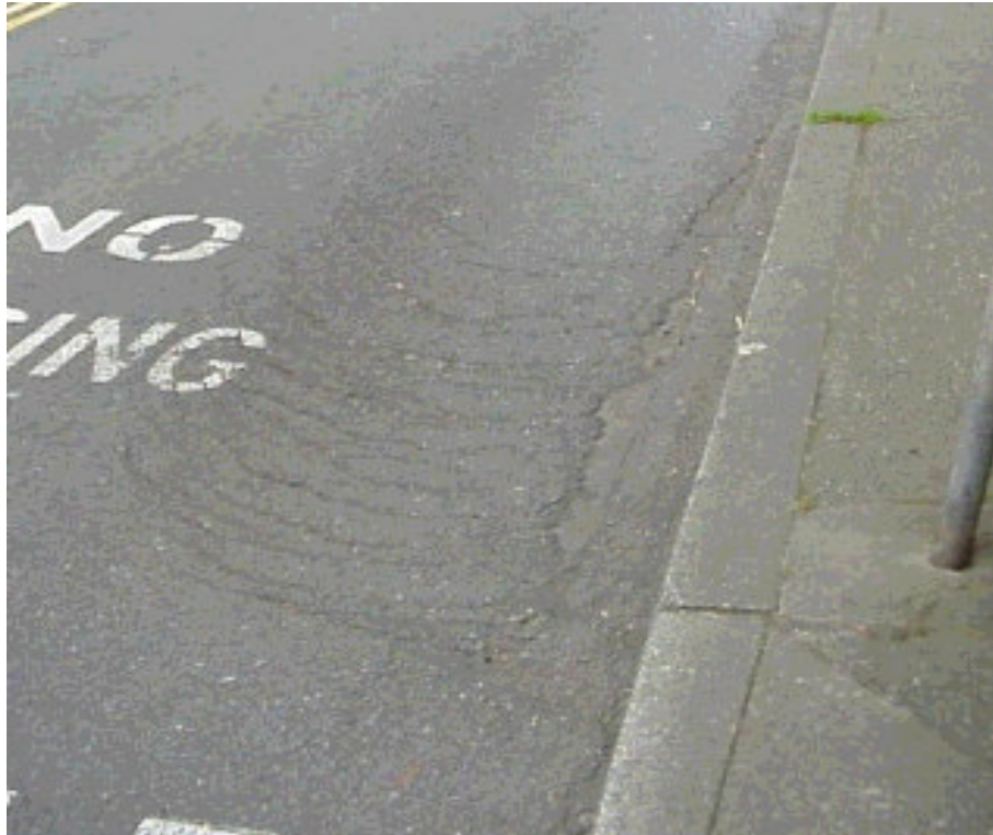
Figure 2.13 – Slippage cracking near to a bus stop, caused by acceleration and braking
