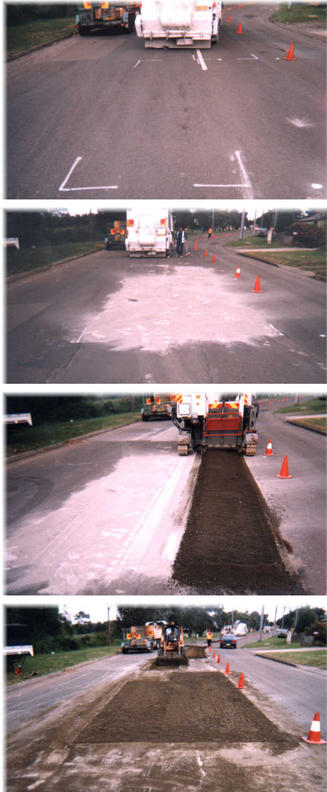
Figure 3.35 – A series of pictures showing the in-situ stabilisation process: before treatment, after stabilisation agent has been placed, mixing of stabilisation agent into soil, after mixing and ready for resealing.
