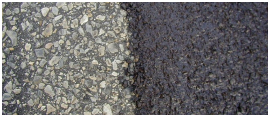
Figure 3.31 – A view of a newly applied slurry surfacing (on the right), compared to the old surfacing
