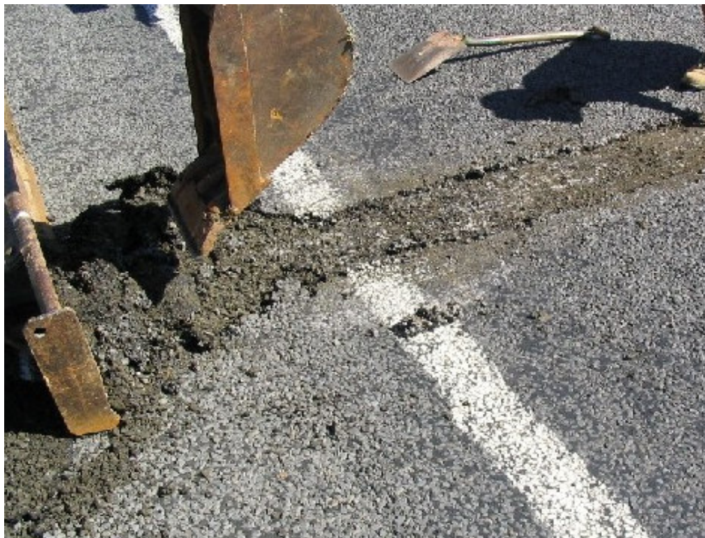
Figure 4.4 – Trenching Part 1:
