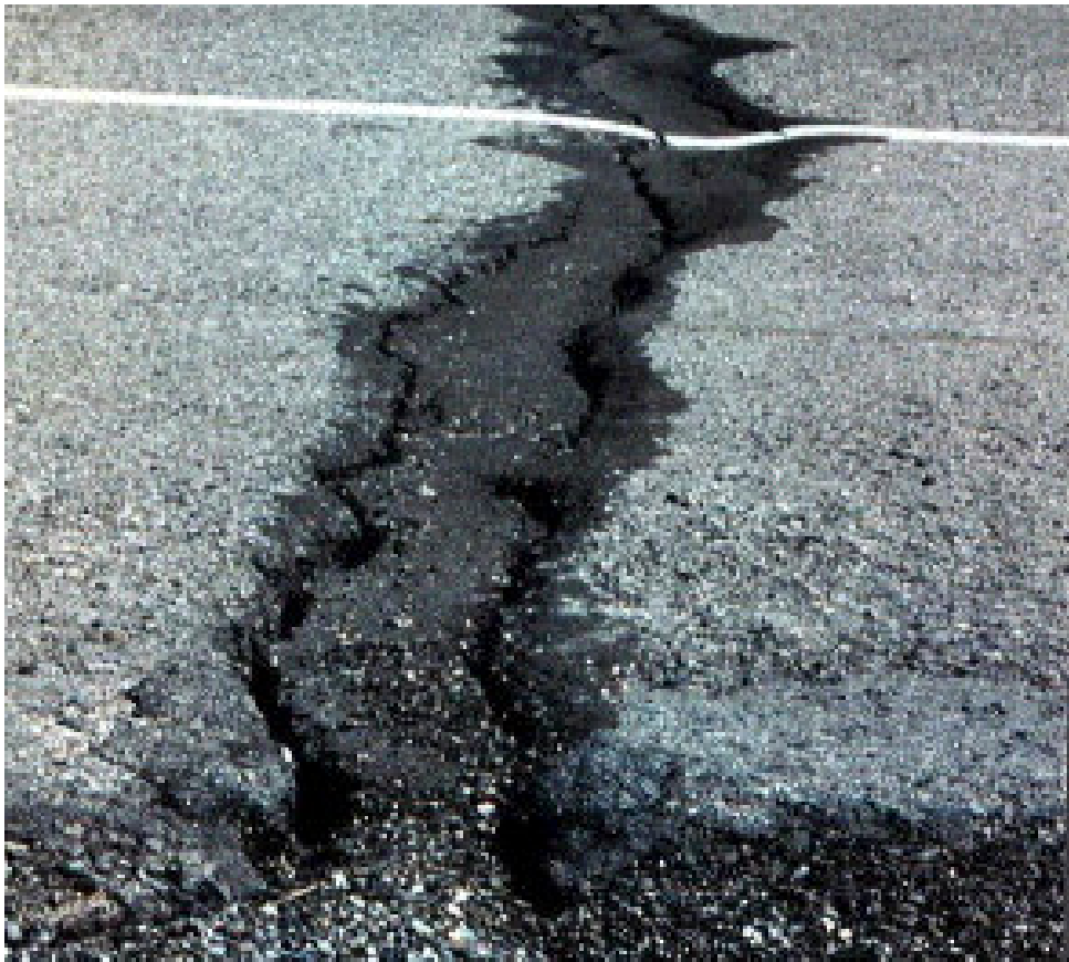
Figure 2.8 – Cold temperatures led to volume change of the pavement materials, and resulted in ‘thermal’ cracking
