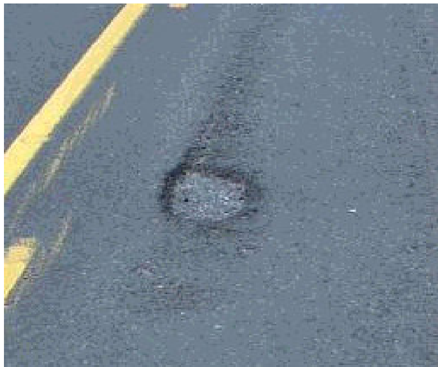
Figure 2.17 – Potholes:
