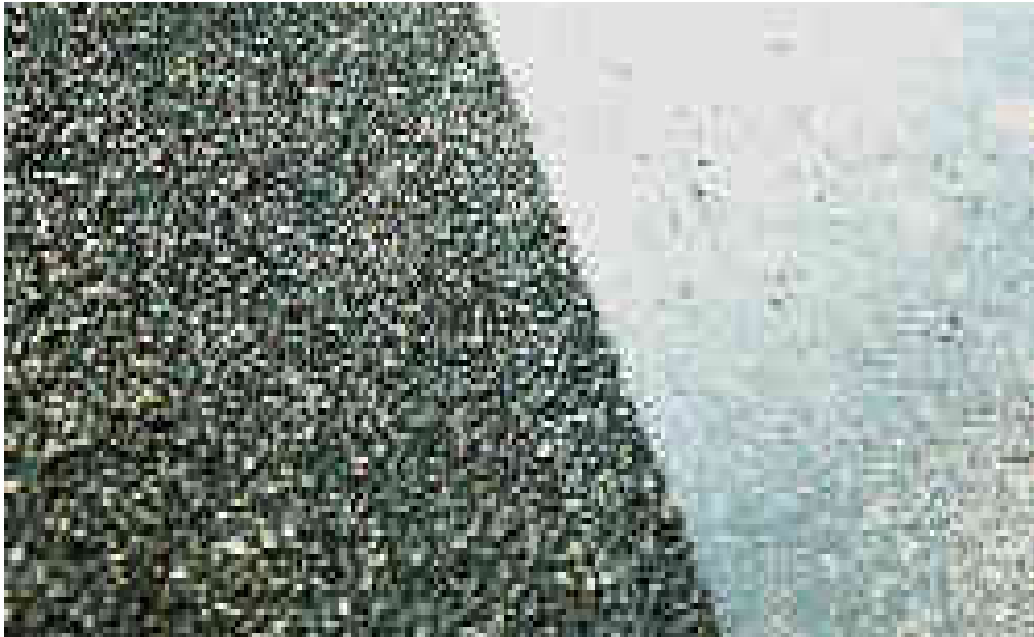
Figure 3.38 – A picture showing a surface before water retexturing (on right) and after water retexturing (on left), showing the large increase in surface texture
