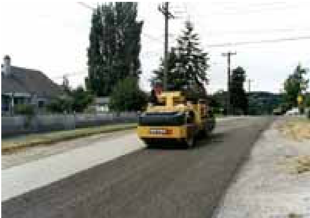
Figure 3.28 – Resealing:
