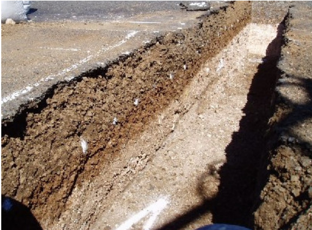
Figure 3.12 – A trench in a pavement, enabling the structure to be easily seen
