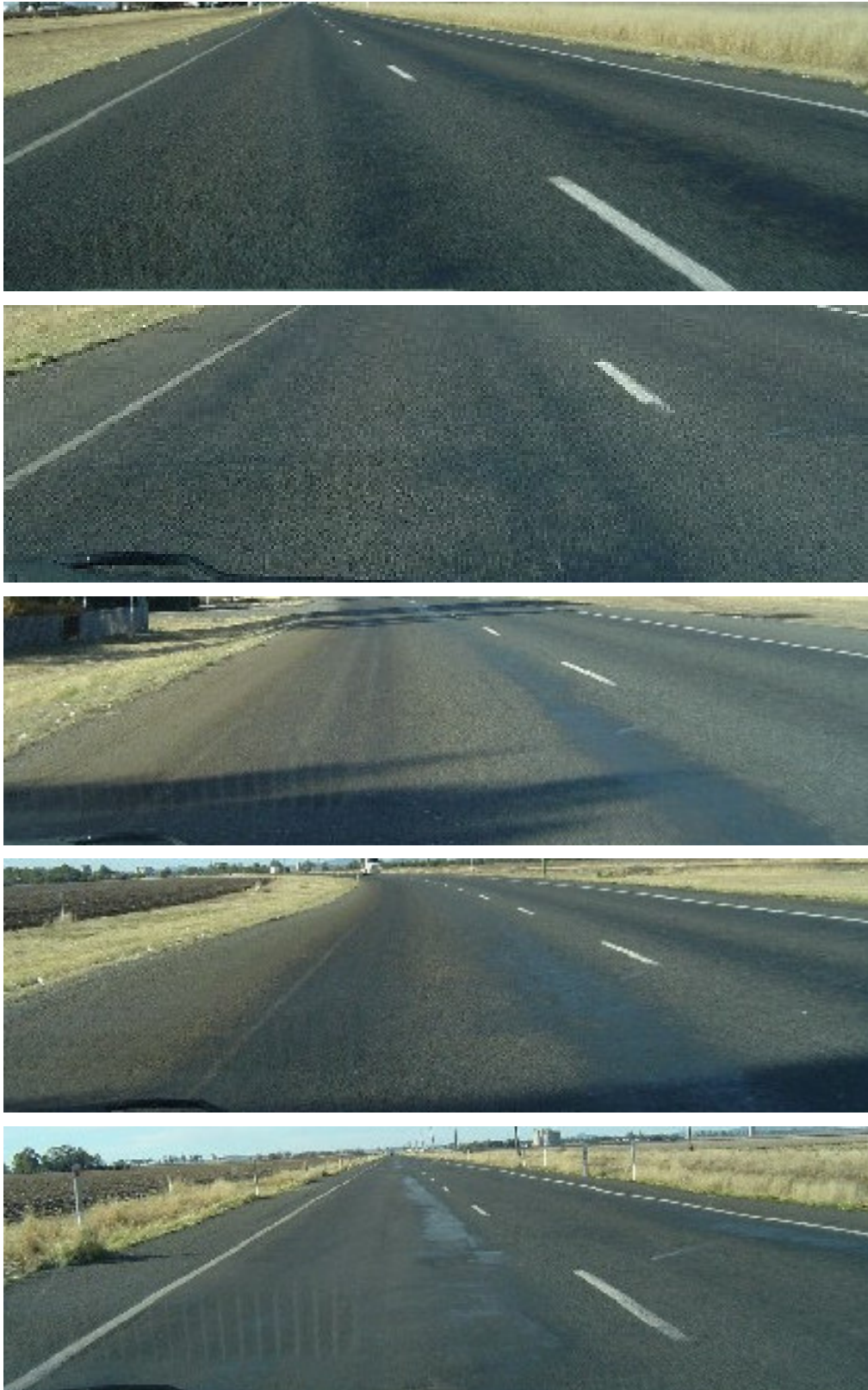
Figure 4.7 – A series of pictures illustrating the variability of bleeding along the section
