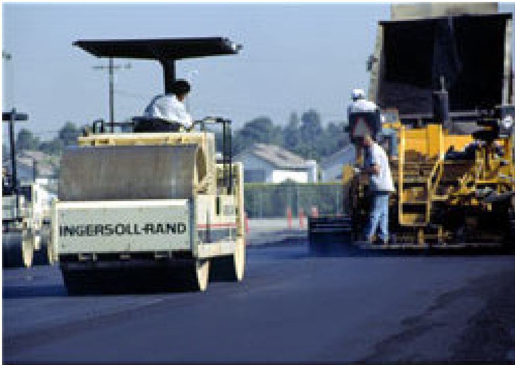
Figure 3.34 – Two views of asphalt overlays being carried out, showing the placement machines and rollers
