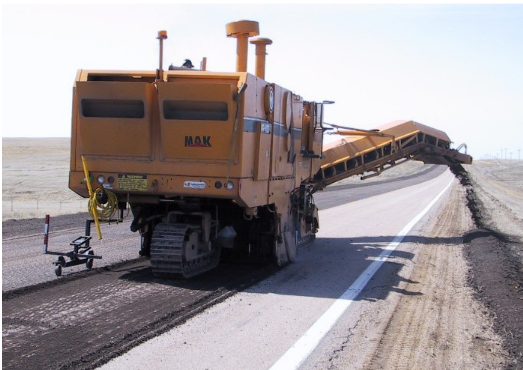
Figure 3.33 – Milling of a surfacing, with the material being deposited along the shoulder
