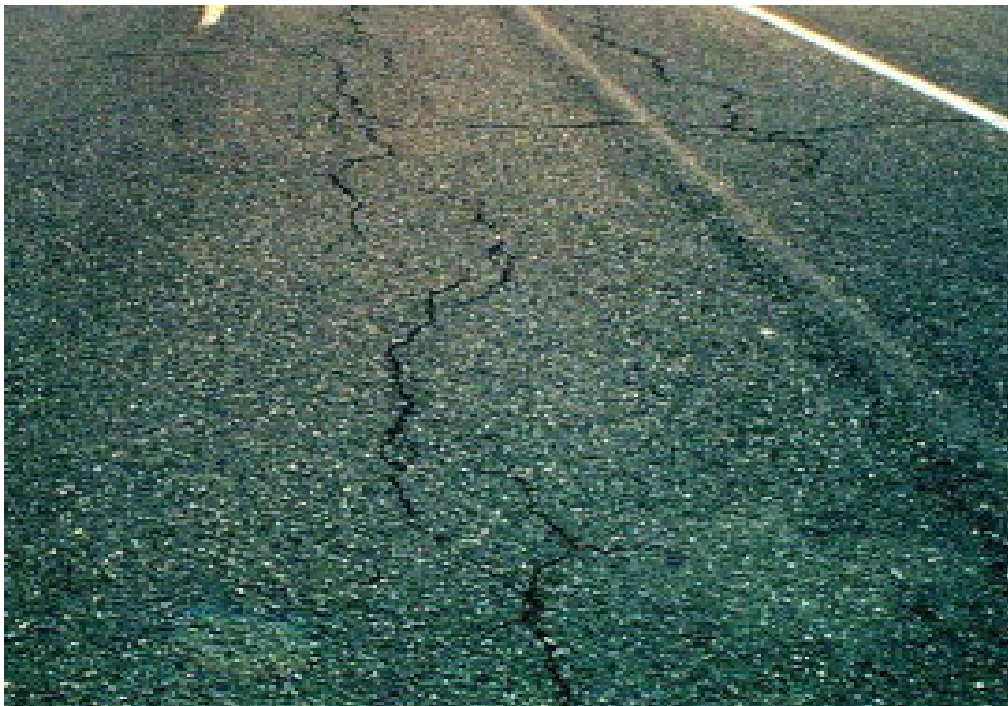
Figure 2.12 – Longitudinal cracking:
