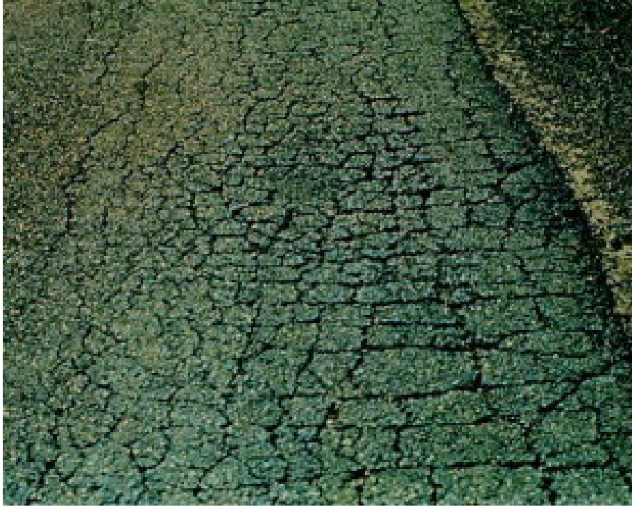
Figure 2.10 – Severe structural cracking, allowing easy moisture entry into the pavement
