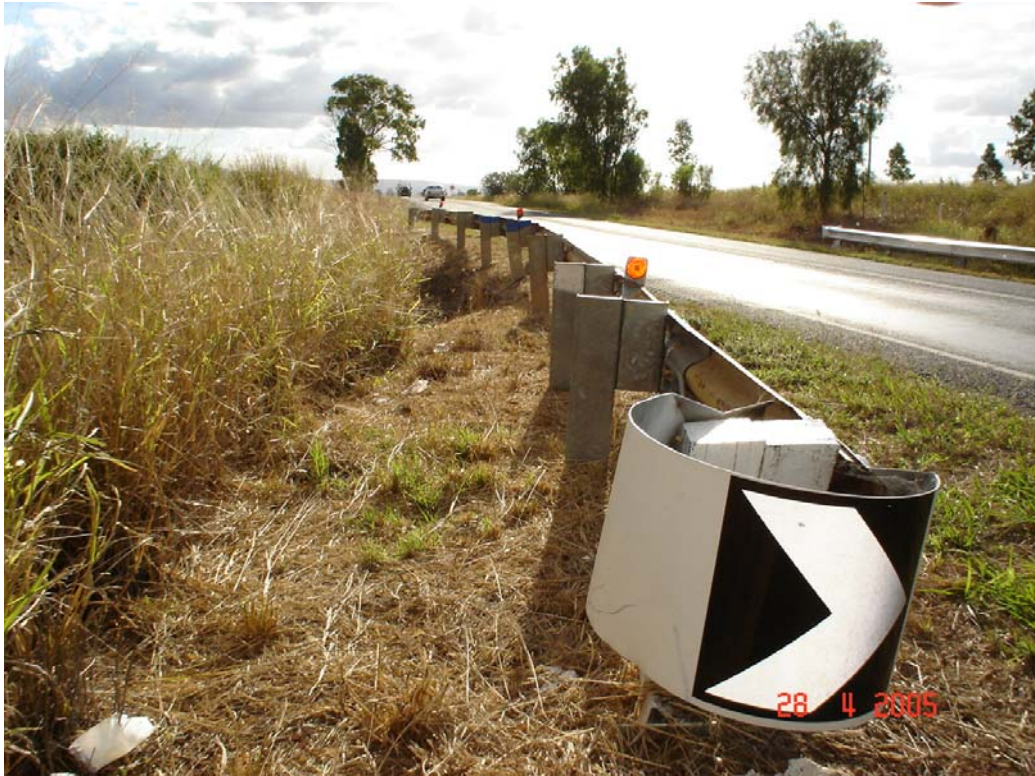
Figure H7 – Noncompliant and damaged guardrail, Gatton Helidon Road. April 2005.
