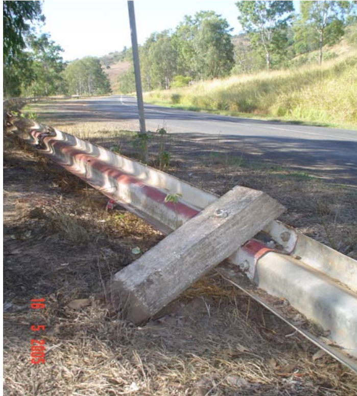
Figure 4.2 – Substandard Guardrail - Rotten Timber Post causing rail to rotate and collapse. (Forest Hill – Fernvale Road, 2005)
