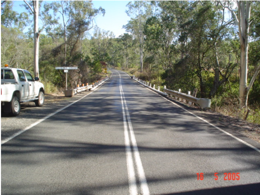
Figure H1 – Noncompliant bridge approach and bridge rail, Esk Hampton Road. May 2005
