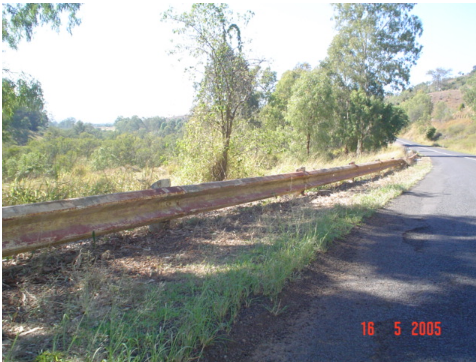
Figure 4.3 – Substandard Guardrail - Poor condition and non compliant height. (Forest Hill – Fernvale Road, 2005)
