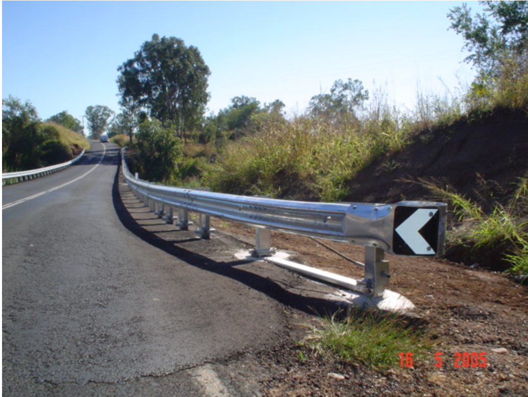
Figure 2.2 – Gating Terminal – Modified Eccentric Load Terminal (MELT) (Forest Hill – Fernvale Road, 2005)
