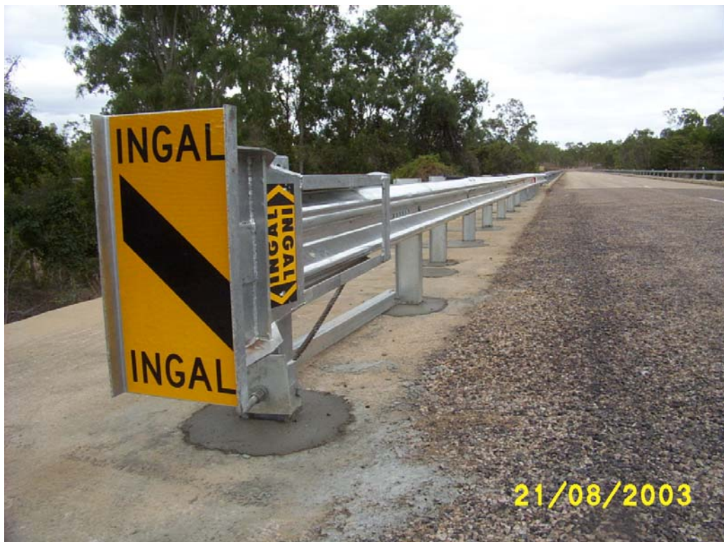
Figure 2.2 – Gating Terminal – Modified Eccentric Load Terminal (MELT) (Forest Hill – Fernvale Road, 2005)
