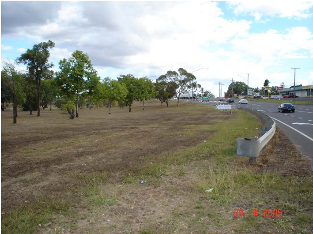
Figure 7.2 – Guardrail identified for removal. No hazard within vehicle clear zone. (Gatton – Helidon Road, 2005)
