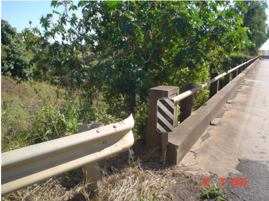
Figure 10.4 – No connection to bridge Forest Hill - Fernvale Road
