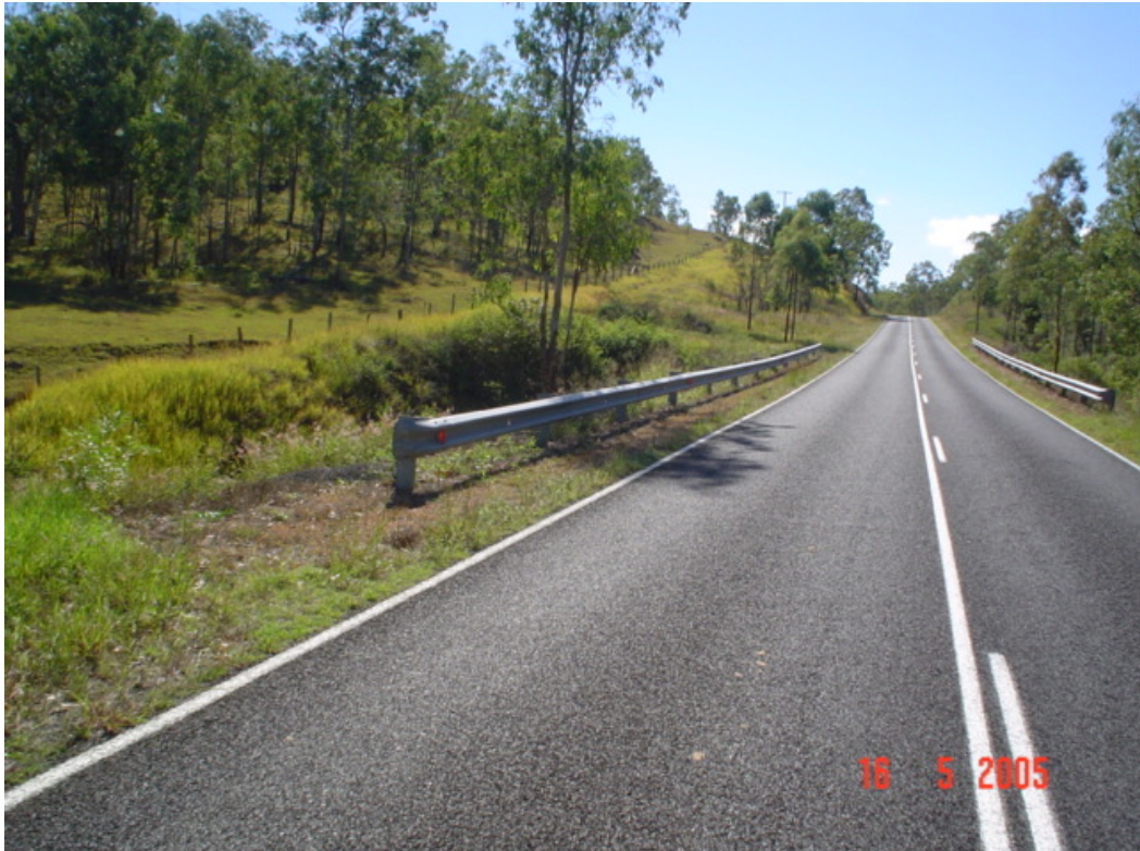
Figure 10.3 – Non conforming guardrail Wivenhoe Somerset Road - Incorrect height and post spacing, no end treatments, and inadequate clear zone behind rail.
