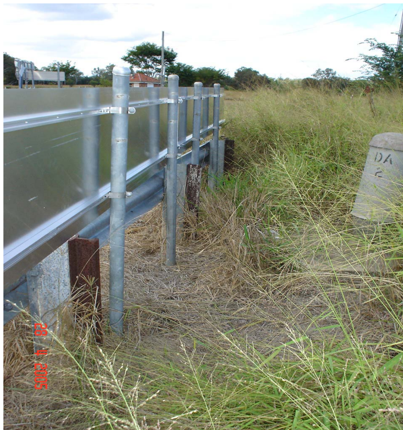
Figure H8 – Substandard posts, Gatton Laidley Road. April 2005.
