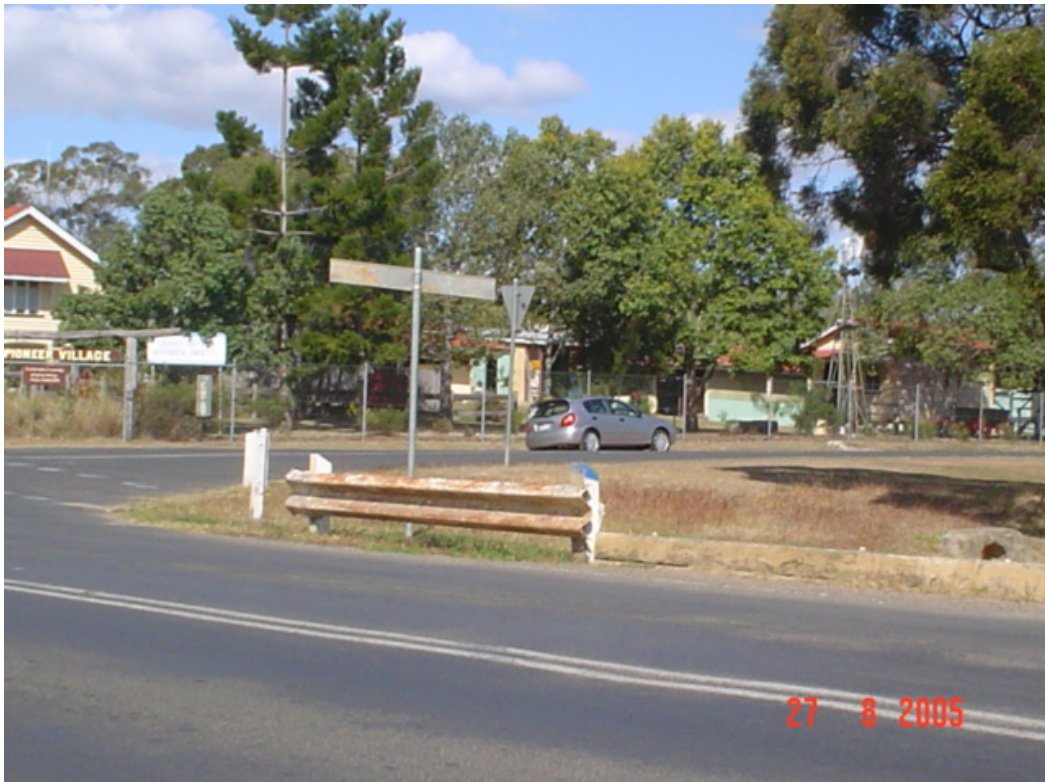
Figure 10.1 – Typical bridge approach rail Rosewood Laidley Road
