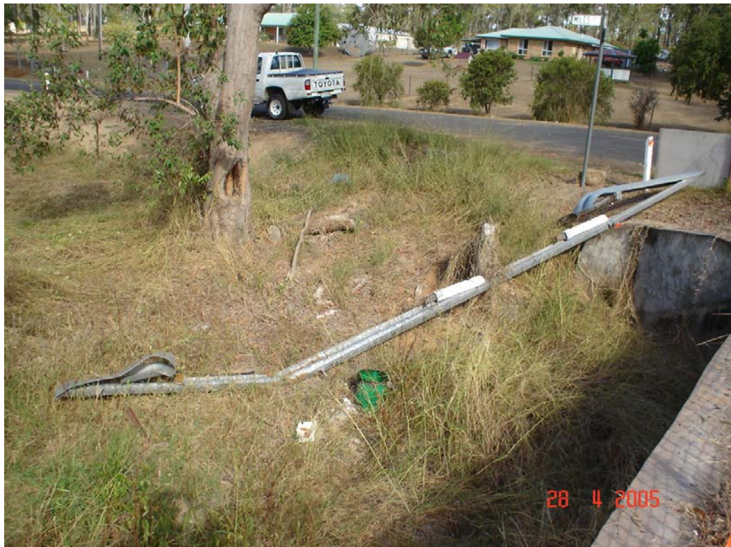
Figure 7.4 – Damaged guardrail due to vehicle collision. (Gatton – Laidley Road, 2005)
