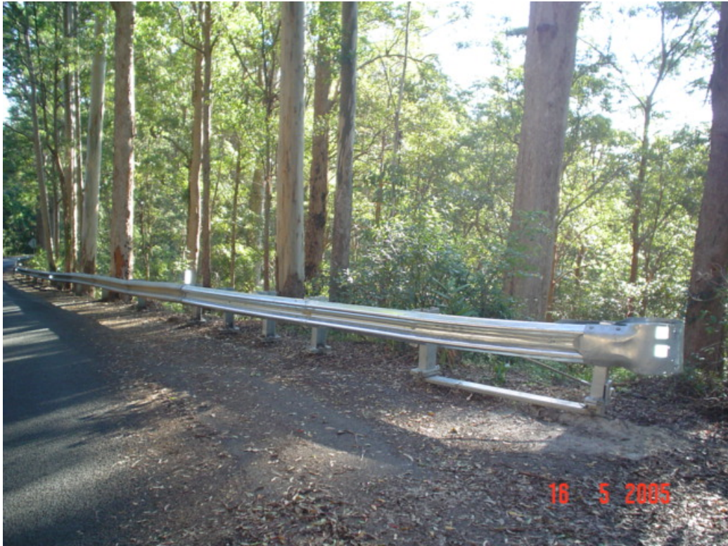
Figure H9 – Trees and steep slope within clear zone of MELT, Mt Glorious Road. May 2005.
