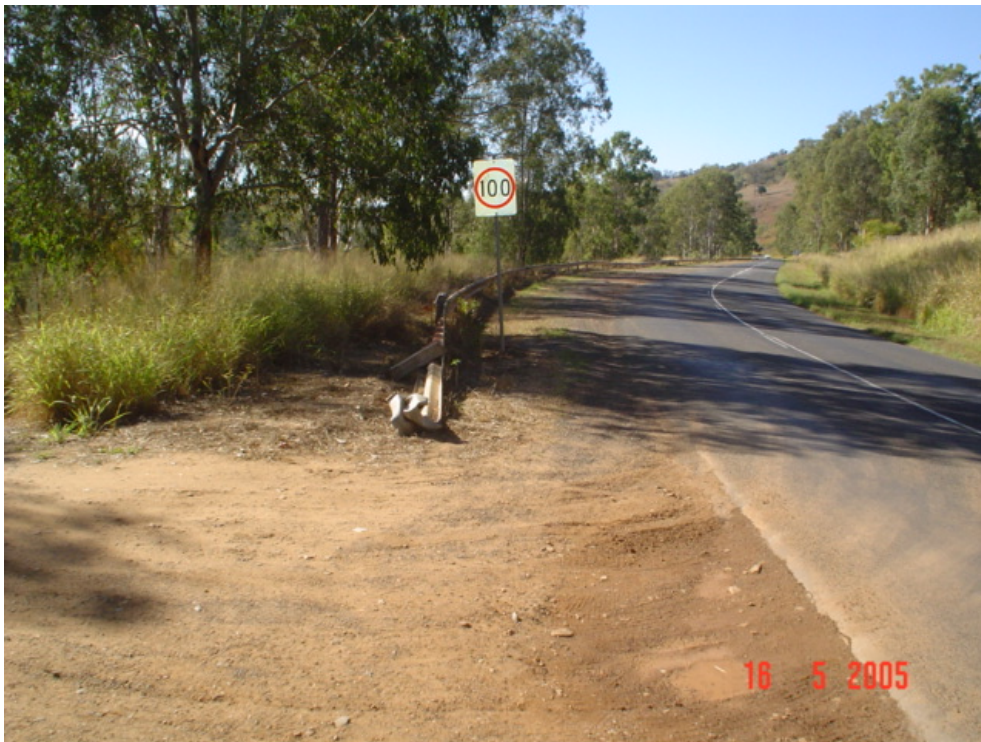
Figure 4.1 – Substandard Guardrail - Damaged and generally in very poor condition. (Forest Hill – Fernvale Road, 2005)
