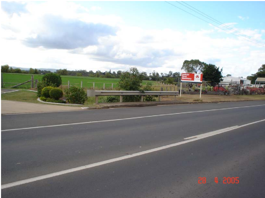
Figure 10.2 – Non conforming guardrail Gatton Helidon Road - Incorrect height and length, no end treatments, incorrect post spacing and inadequate clear zone behind rail
