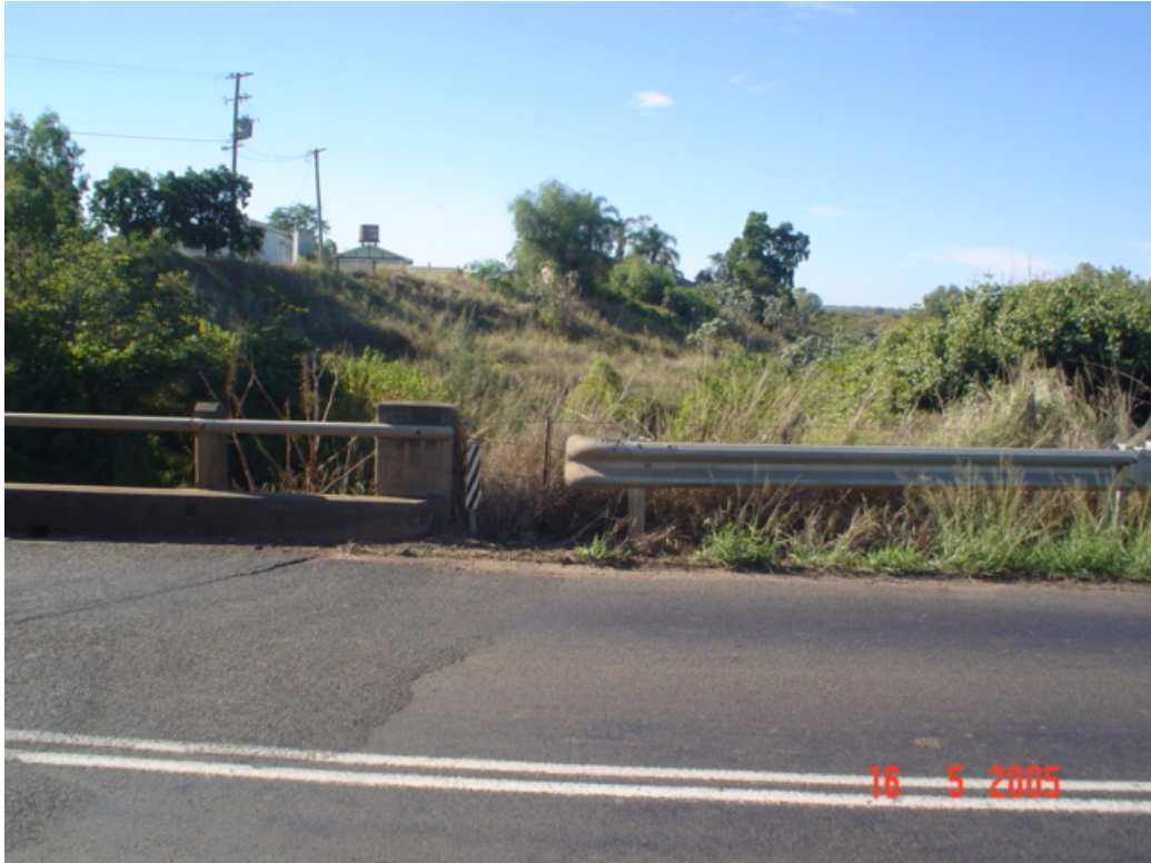
Figure H3 – Noncompliant bridge connection, Forest Hill Fernvale Road. May 2005
