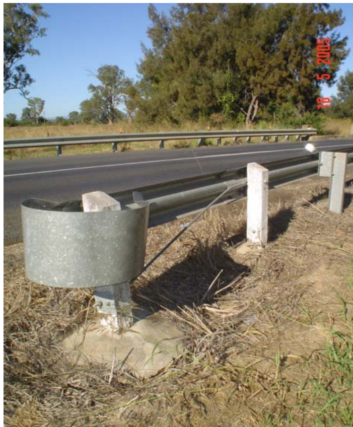
Figure H2 – Noncompliant End Treatment, Forest Hill Fernvale Road. May 2005
