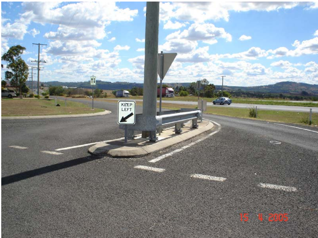
Figure H10 – Noncompliant guardrail and end treatments, Warrego Highway Service Road. April 2005
