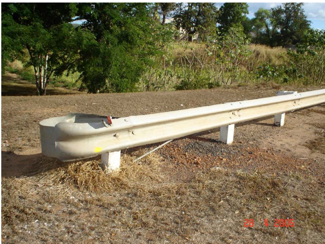
Figure H6 – Noncompliant end treatment, Gatton Helidon Road. April 2005
