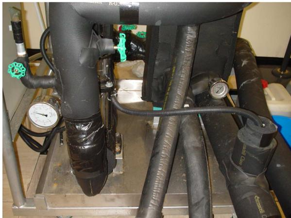
Fig. 5.5 External Chiller Water Pan
