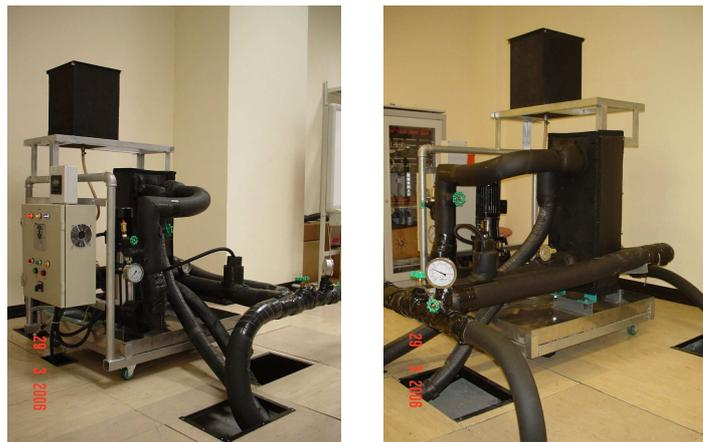
Fig 1.6 Two views of the External Chiller
